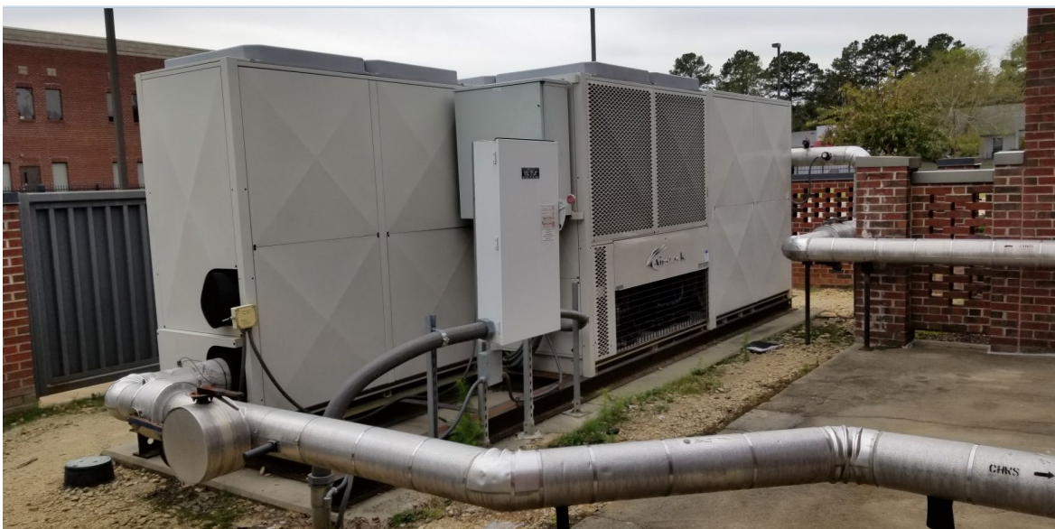
Figure 8 – Air Cooled Chiller in Mechanical Yard
