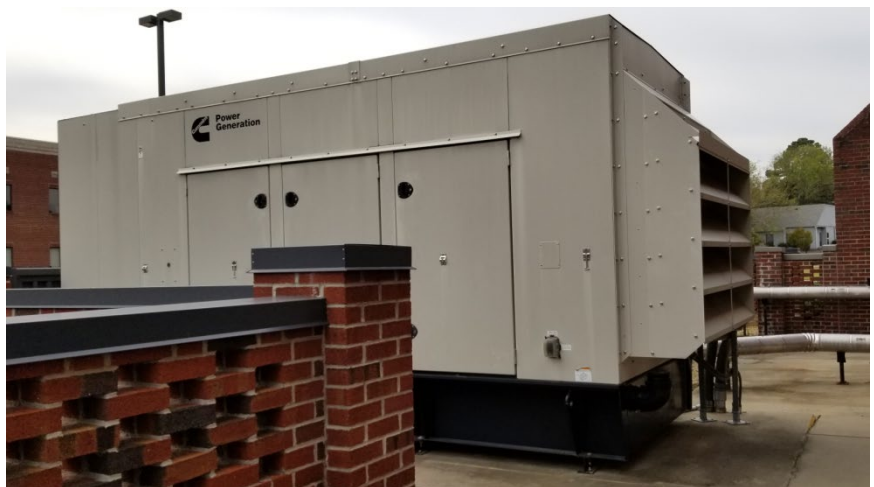
Figure 10 – Existing Generator
