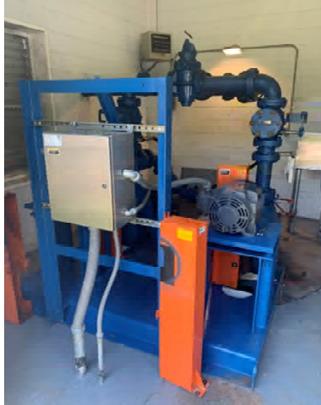
Minor corrosion on piping
