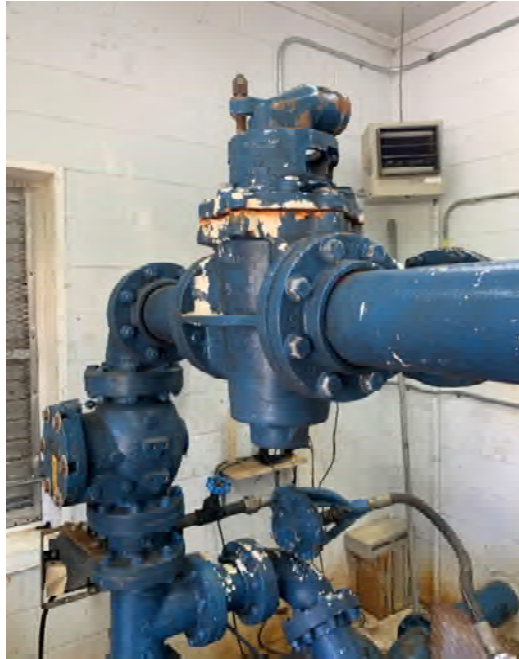
Corrosion on piping and valves
