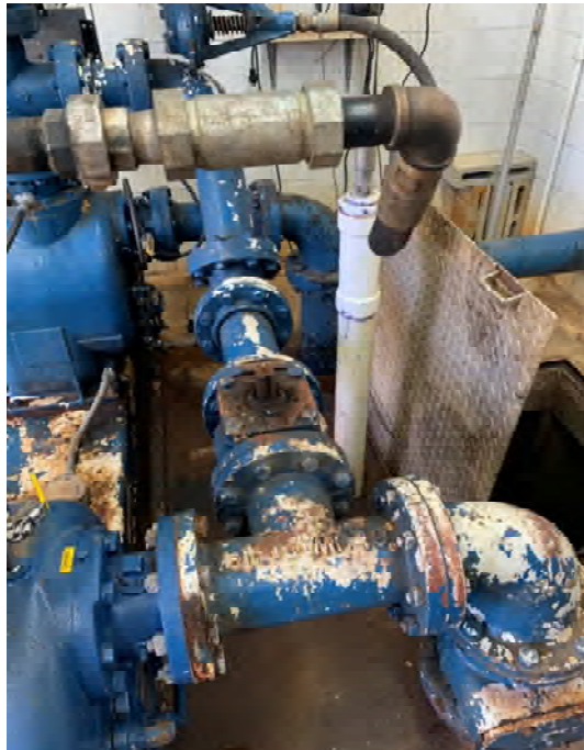
Corrosion on piping and valves
