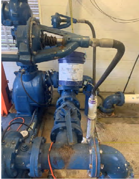
Corrosion on piping
