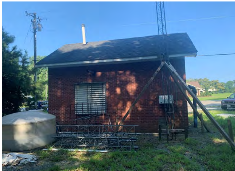
Wet well vent rusted comm tower base. Safety concern.
