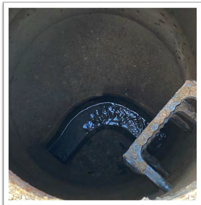
SMH 026913, King Street in Falcon. Manhole in good condition.
