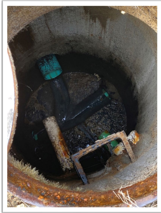
MH FID 30, BRINKLEY DRIVE, GOOD.
