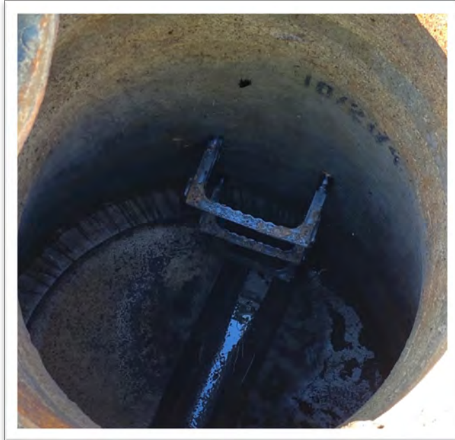
SMH 027930, Main Street in Godwin. Manhole in good condition.
