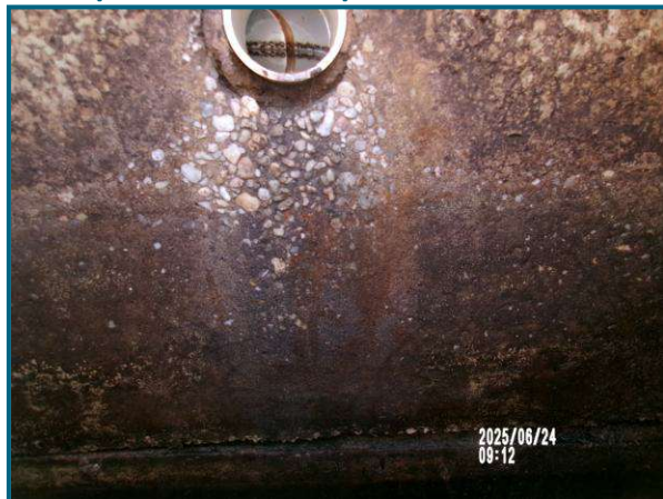
P7. Septic Tank Inlet Pipe
