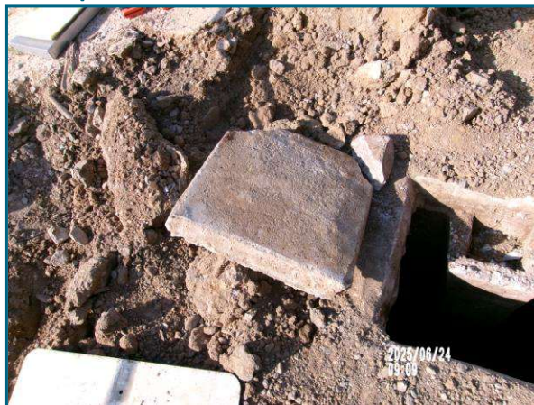
P4. Septic Tank Outlet Lid
