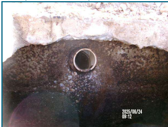
P8. Septic Tank Interior
