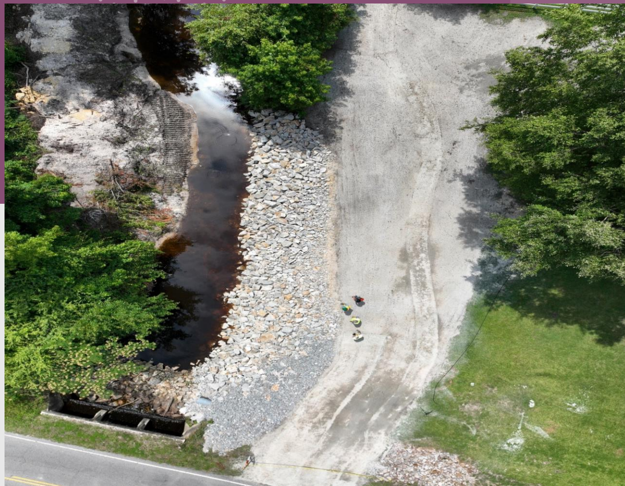
After Streambank Stabilization
